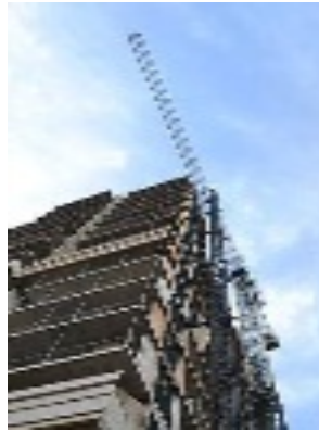
Condo construction in Canada
